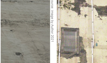
Surface cracking (and spalling) visible on the concrete surface.
