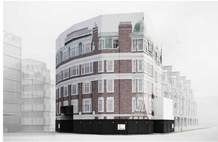
Building wrap and dehumidifiers to dry out the building initially. (Source: embracebuildingwraps uk)
